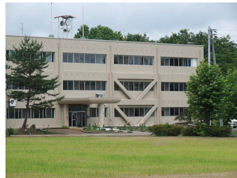
(c)耐震補強の状況
