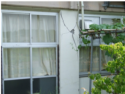
(c)柱の損傷
