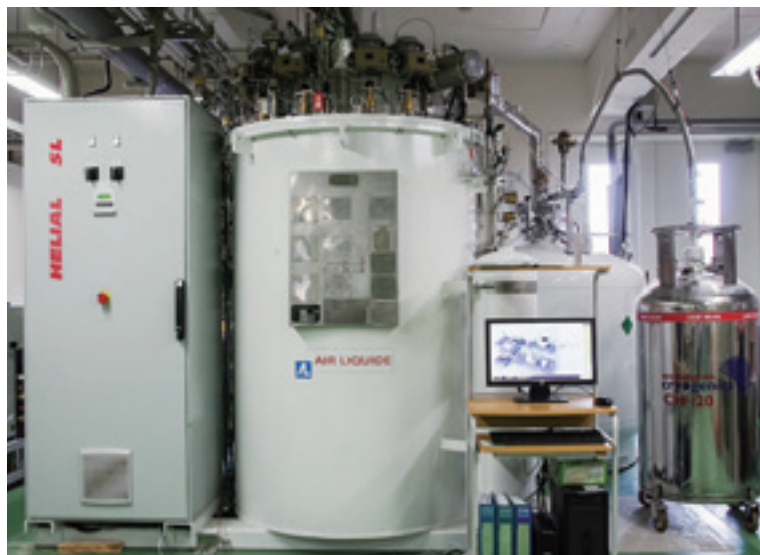
Fig. 1: Helium liquefier in CL
